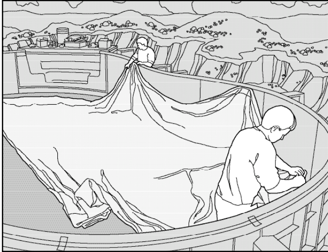
2. Unfold the liner with the arrows pointing at the shallow end corners. Note plywood and 2x4 with strip to hold liner during install.
