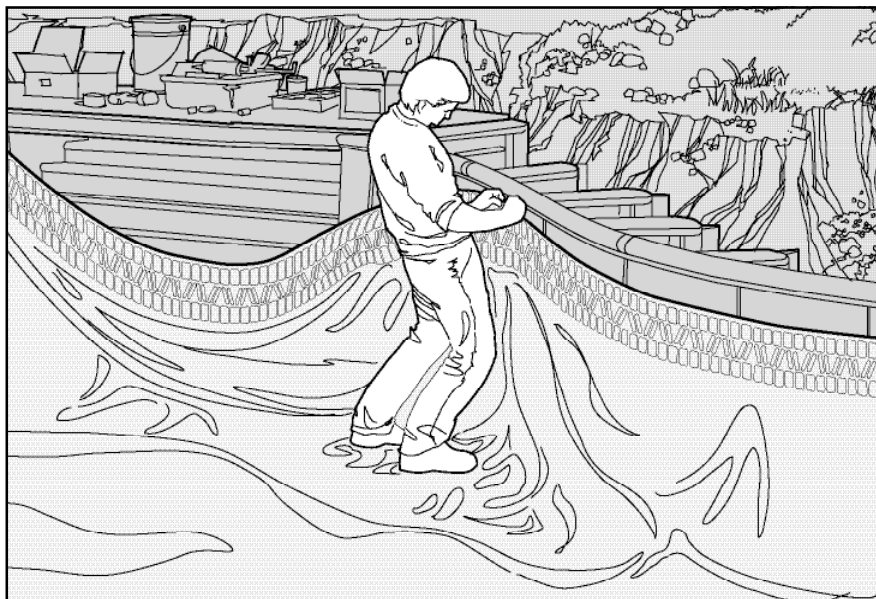
3. Unfold the rest of the liner toward the deep end of the pool.
